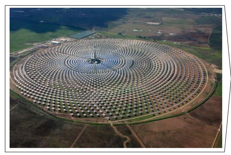
Allowing for very high HTF operating temperatures (565 to 1000°C), depending on which technology is used
