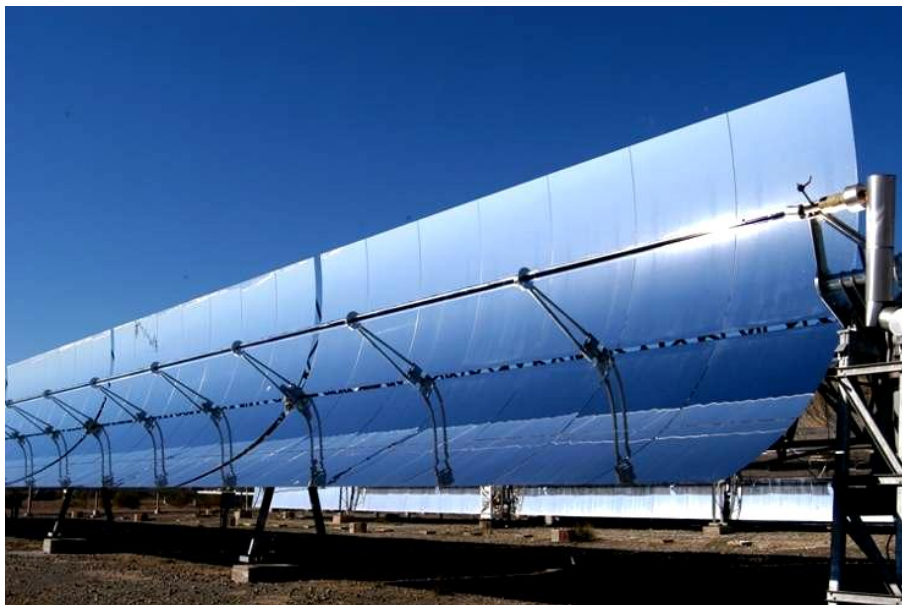
Figure 2.4 - EuroTrough Parabolic Trough Collector.
