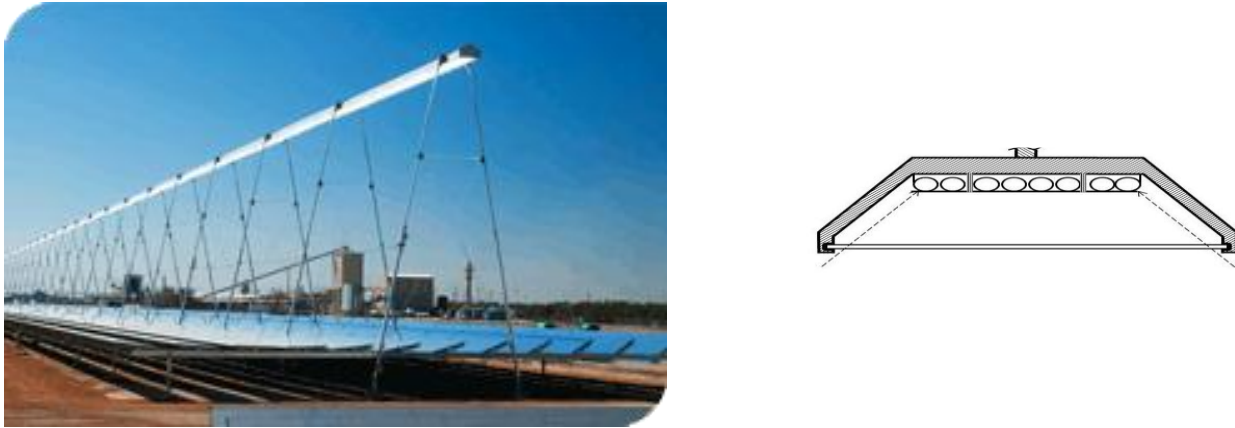
Figure 2.8 - Example AREVA Solar “CLFR” field showing the fixed receiver and internal receiver structure.
