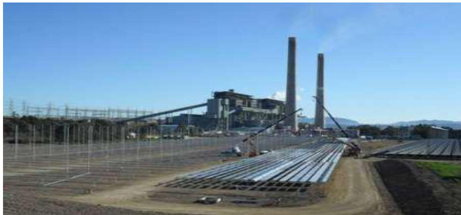
Figure 2.35 - Liddell solar field booster for the Liddell coal-fired power plant. (Source: AREVA - Liddell Solar Thermal Station.
