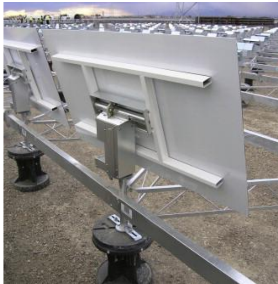
Figure 2.19 - Mounted heliostats of the Sierra SunTower heliostat field ( http://www.sciencedirect.com/science/article/pii/S0038092X10000216 ).
