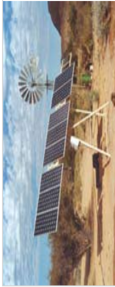
A Solar Water Pump uses solar photo-voltaic panels to provide energy for pumping water for livestock and domestic use.
