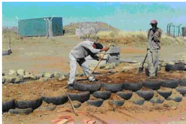
Tyre wall construction
