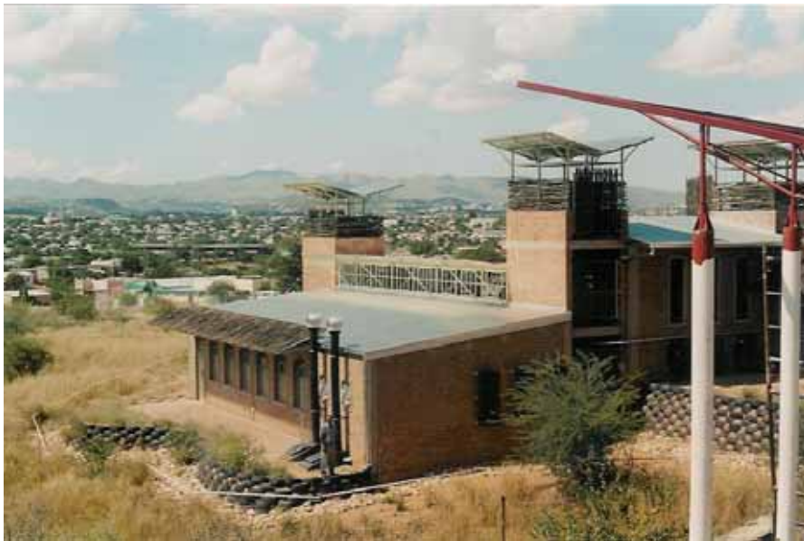
Clerestory windows for ventilation and light
