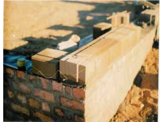
construction with stabilised soil blocks
