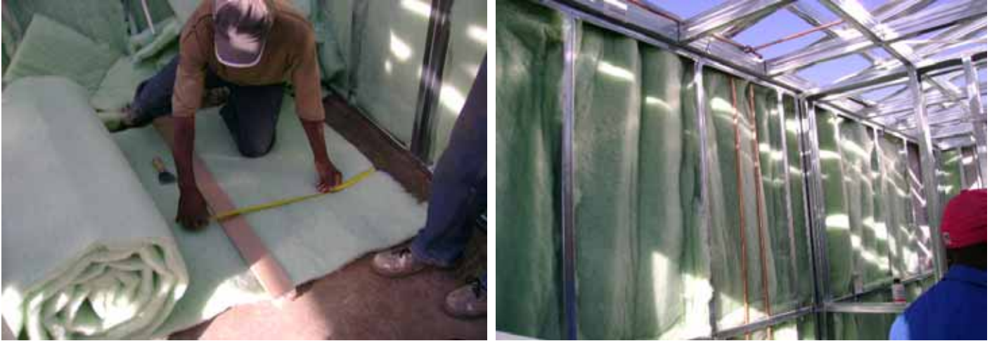
Insulating walls and roofs
