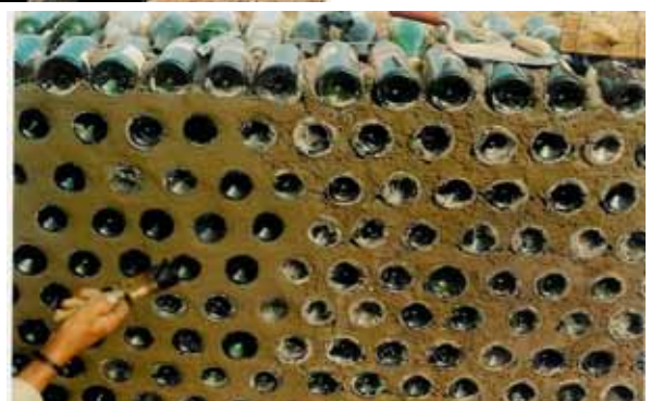
Alternative wall construction materials (building rubble in gabions, tyres, bottles)
