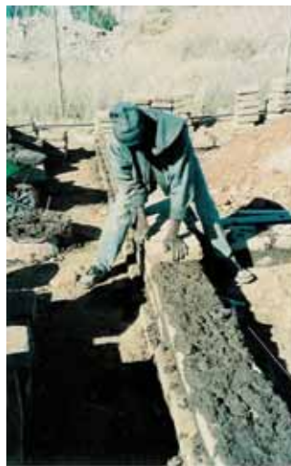
Rammed earth foundation and clay wall construction
