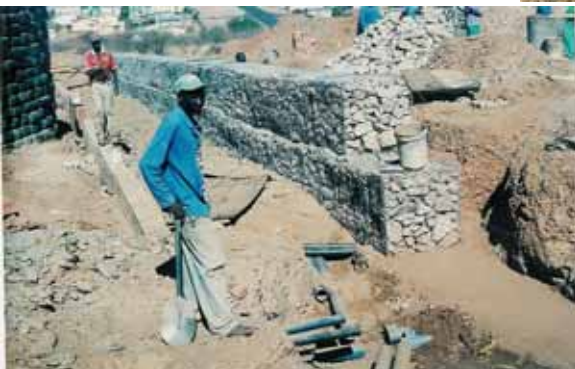
Alternative wall construction materials (building rubble in gabions, tyres, bottles)
