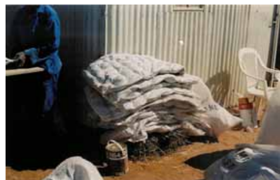
Ceiling made from reed, old plastic bags and wool filling
